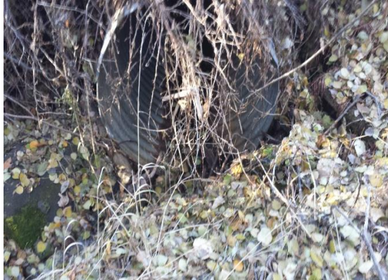
Photo 12: Crossing 2 culvert outlet.
