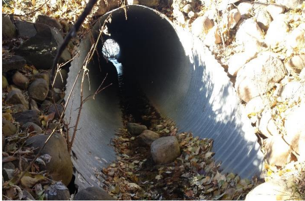
Photo 5: Crossing 1 culvert inlet.
