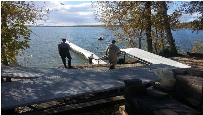
FIGURE 6: INSTALLING OF A DOCK (SOURCE: SUMMER VILLAGE)
