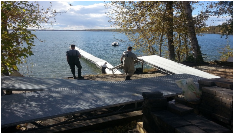
FIGURE 6: INSTALLING OF A DOCK (SOURCE: SUMMER VILLAGE)
